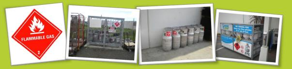
Note: For any ignition sources (IE: electrical fittings, lights, alarms etc.) within these zoned areas you are required to obtain an electrical certificate of compliance issued by a qualified electrical inspector.
